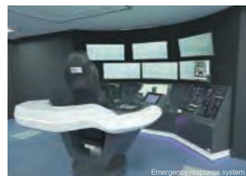
Emergency response system
