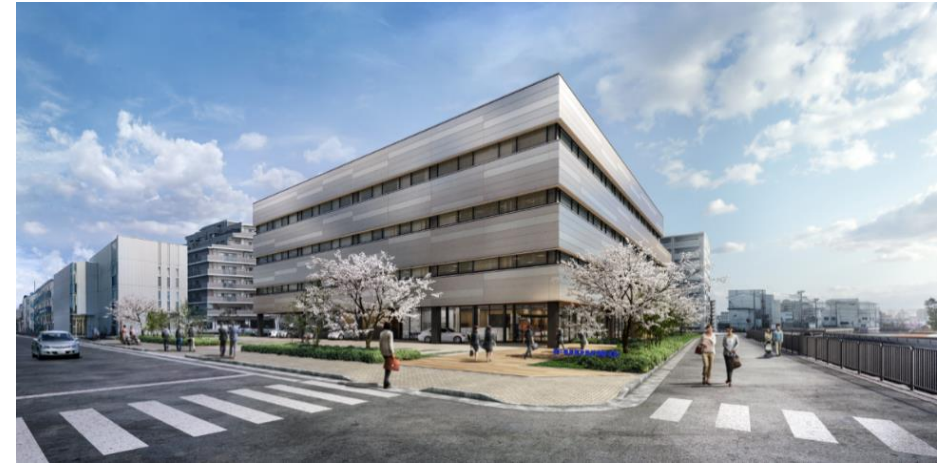
New R&D Work Space (completion scheduled September 2021)
