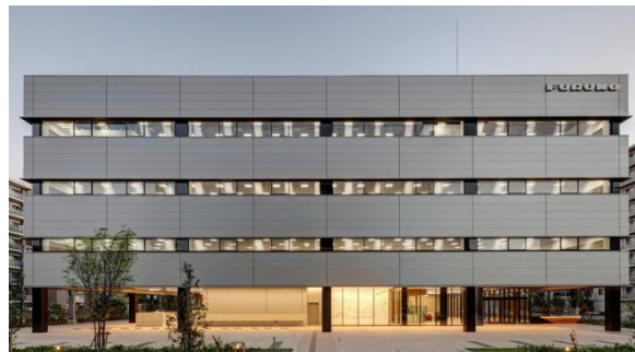
New R&D Building SOUTH WING
