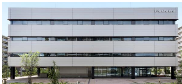
R&D Building SOUTH WING
