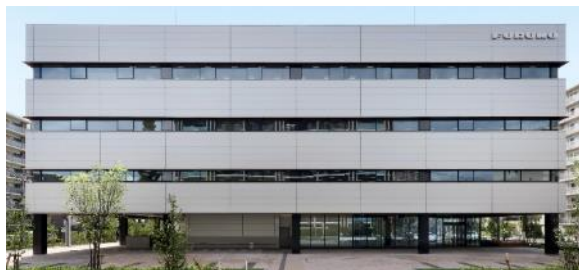
New R&D Building SOUTH WING
